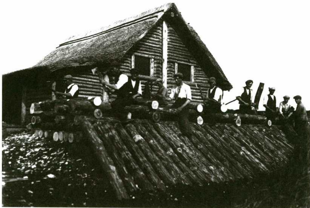
Fig. 2: Biskupin 1937. The expedition carpenters building a fragment of the breakwater reconstruction. Photo Biskupin Museum Archives.
