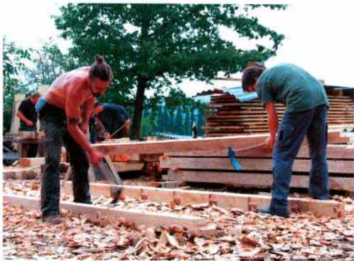
Abb. 4: Alle Pfosten und Sparren wurden von Hand behauen, alle Bretter von Hand gehobelt. – All posts and rafters were axed, all planks planed by hand.
